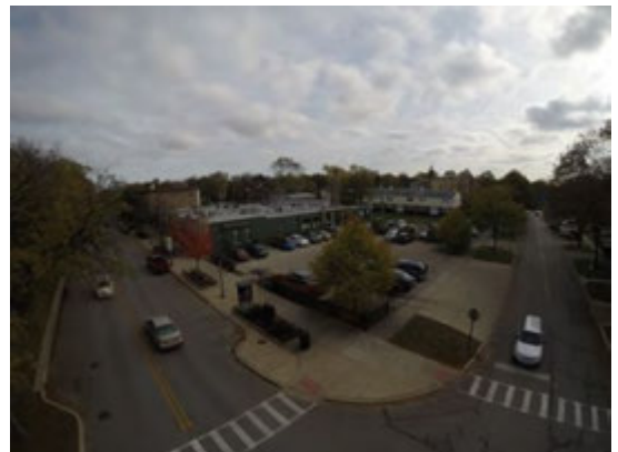
Corner view, looking southeast
